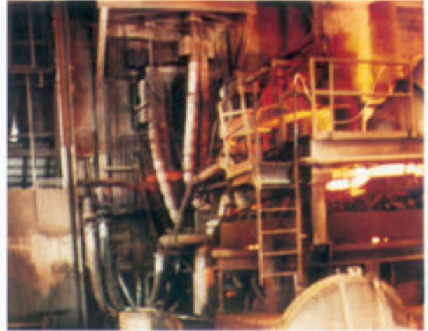
GSM Water Feed/Return Lines can range from 3" to 8" inside diameter.
